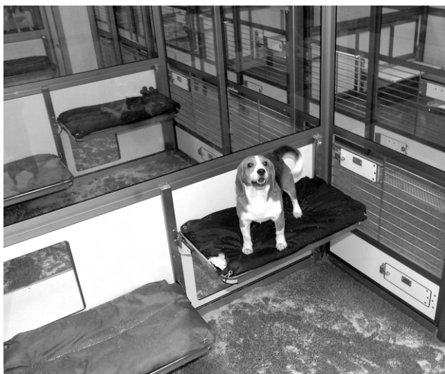
Figure 30.3 Glass panels between pens can improve overall visibility and reduce levels of barking. (Reproduced with permission of Astra Zeneca.)
