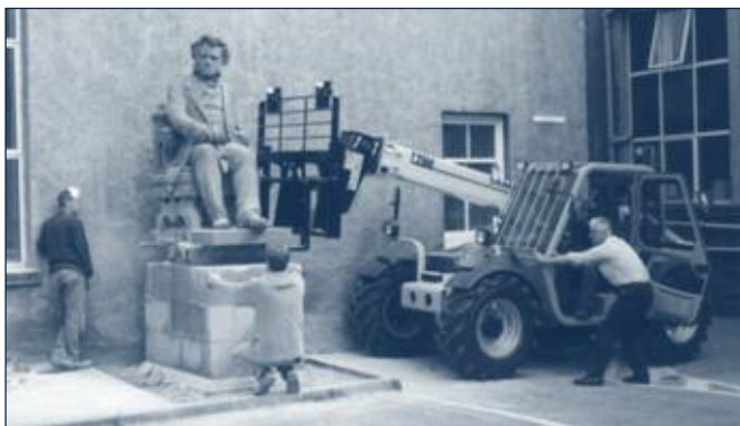
Lifting from the plinth.
