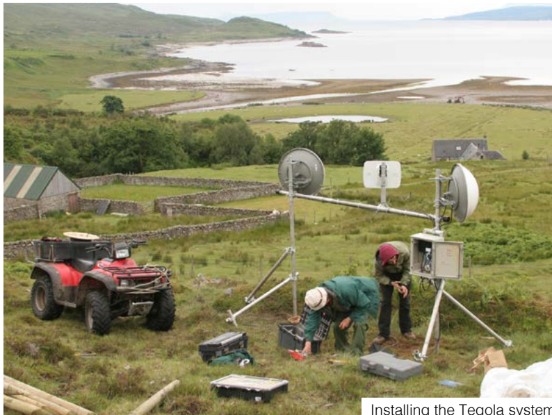
Installing the Tegola system
