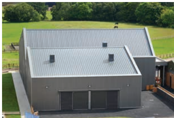
The new EDSCCU
